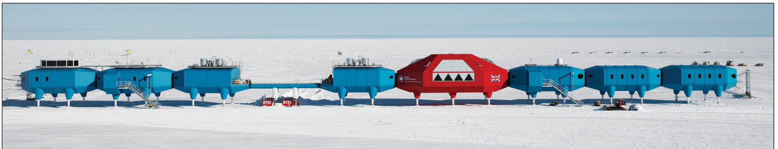
The Halley VI British Antarctic Research Station, which is a relocatable science research station incorporating biophilic design. See more about it at hbarchitects.co.uk/halley-vi-british-antarctic-research-station/
